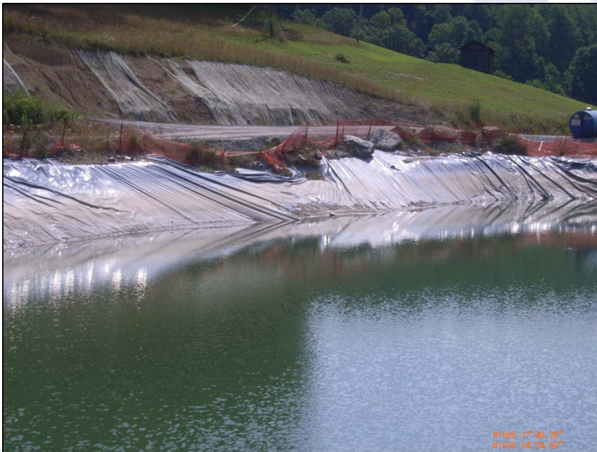
Bank failure under liner
